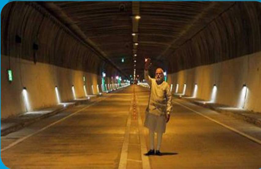
Chennai Nashri Tunnel
